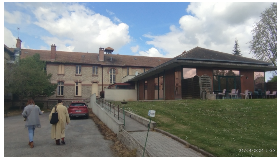
Extension n°2 cuisine restaurant
